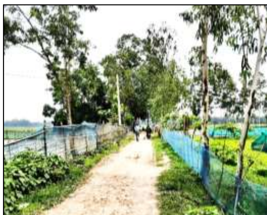
MADH-R-03: Improvement of Road by RCC From Fazlul Commissioner Dampara Madhupur JICA road to Pundhura JICA road via Hobir Bari road including Protection Work at (Ch.20m to 45m, R/S), (Ch.215m to 240m, R/S) & installation of Street Light 45 nos. at Ward no. - 7, Madhupur Pourashava, Tangail. Total Length = 665m.
