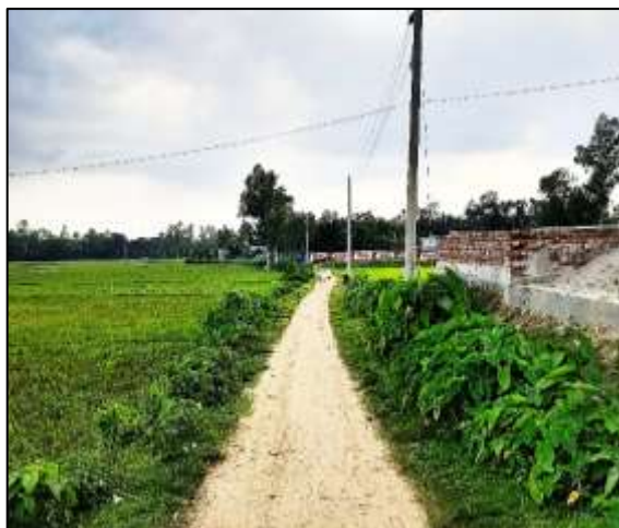
MADH-R-01: Improvement of Road by RCC From Tangail - Mymensingh road (near Vulasha Mour) to Ashura Road (Ch.0.00m to Ch.560.00m) including RCC Cross Drain, Protection Work & installation of Street Light 38 nos. at Ward no.-9, Madhupur Pourashava, Tangail. Total Length = 560m.
