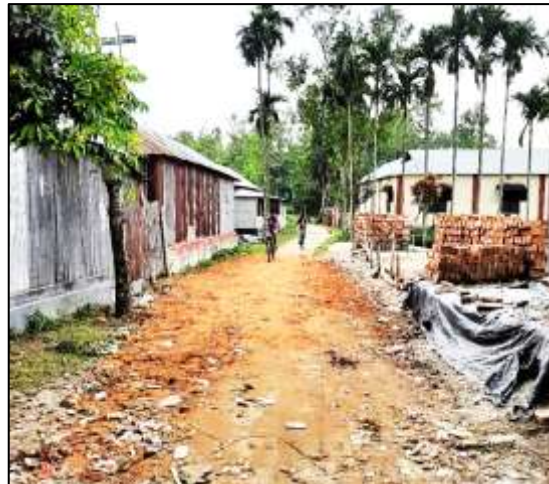
MADH-R-02: Improvement of Road by RCC From Gopalpur road Togor shop to Hobidpur UP road (Bridge) (Ch.0.00m to Ch.690m) including Protection Work & installation of Street Light 47 nos. at Ward no.-9, Madhupur Pourashava, Tangail. Total Length = 690m.
