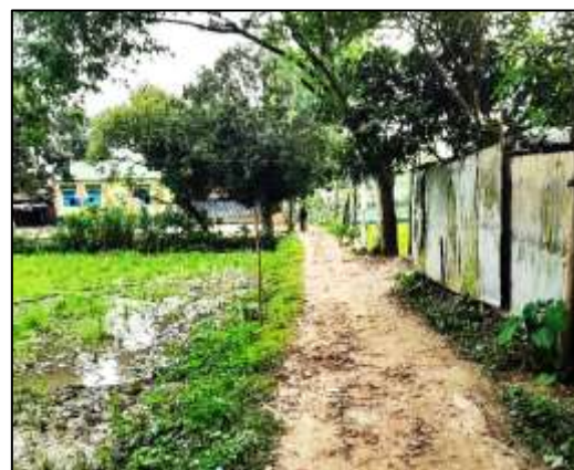
MADH-R-04: Improvement of Road by RCC (a) From Pirujpur road near Biprobati Jalil House to Hazi Bari via Hafiz House Road (b) Link 1: Jalil House road including RCC Cross Drain at Ch. 184m, Ch. 225m, Protection Work installation of Street Light 27 nos. at Ward no.- 4 Madhupur Pourashava, Tangail. Total Length = 395m.
