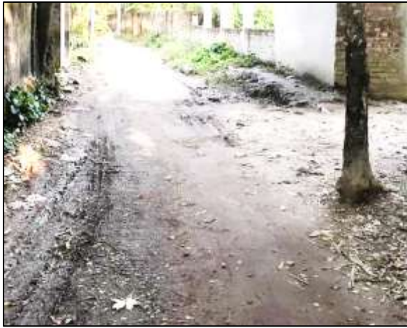
CP-R-144: Improvement of Road by RCC Noyahat from Islam Badi Road to Harala (Ch. 0.00m to Ch. 670m) installation of Street Light 23 nos. at Ward no. - 06 & 04 at Chandanish Paurashava.
