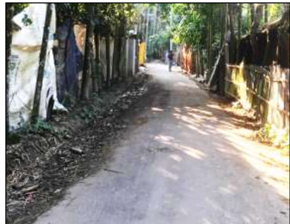
CP-R-241: Improvement of Road by Dense Bituminous Carpeting from BMDF Road via Khanhat to Abdulbari Hat Gachbaria at Ward no. - 09 & 08 Chandanish Paurashava.
