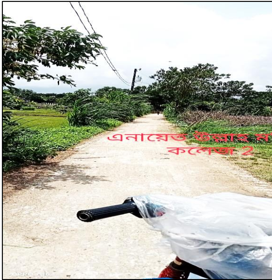
Road-06 + Drain-07, Sonagazi Pourashava
