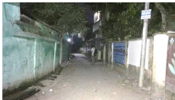
Drain-022, Brahmanbaria Paurashava
