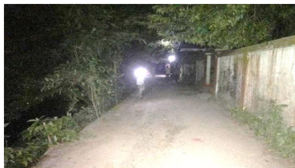
Road-007, Brahmanbaria Paurashava
