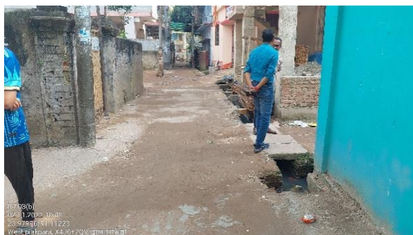
Road-003, Brahmanbaria Paurashava
