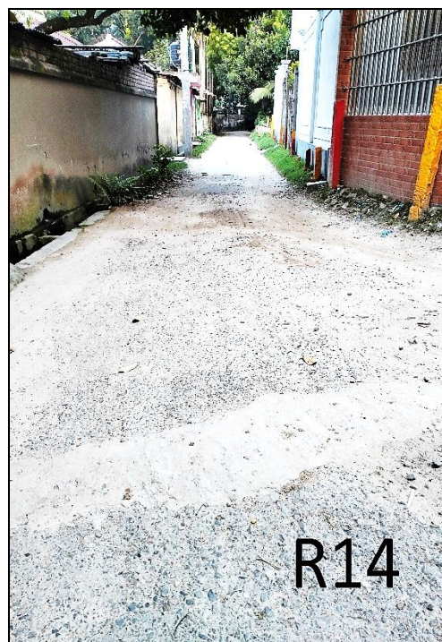
BHER-R-14: Improvement of road by Dense Bituminous Carpeting from Bacchu house to Sadek house road (Taltola road) (Ch. 0.00m to 460m) & installation of Street Light 16 nos. at Ward no. - 8, Bheramara Paurashava, Kushtia. Total Length = 460m.
