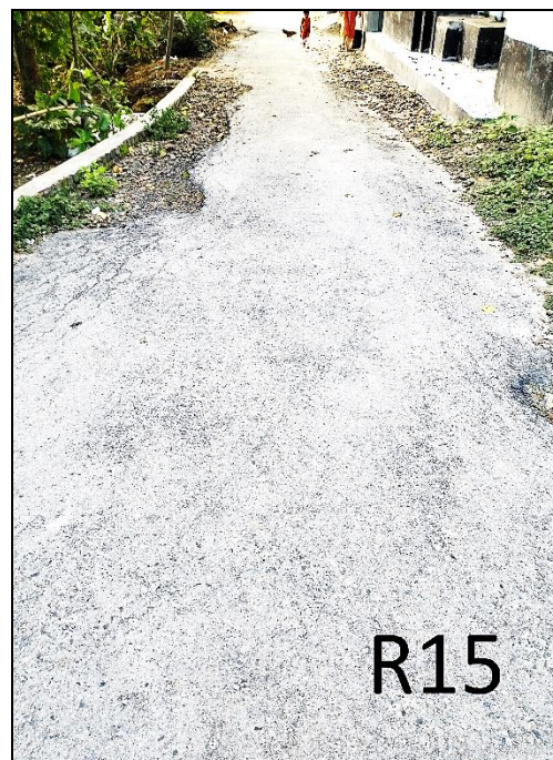
BHER-R-15: Improvement of road by Dense Bituminous Carpeting from Pragpur road to Eidgah road (Ch. 0.00m - 375m) & installation of Street Light 14 nos. at Ward no. - 5 & 7, Bheramara Paurashava, Kushtia. Total Length = 375m.
