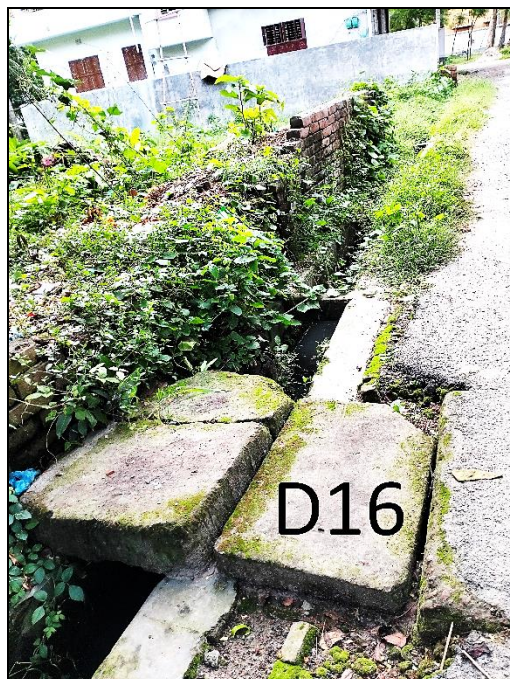
BHER/D-16: Construction of RCC Drain from existing drain near H/O Khairul Councilor to Hisna River (Ch. 0.00m to 400m) at Mothpara Ward No. - 08, Bheramara Paurashava, Kushtia. Total Length = 400m.
